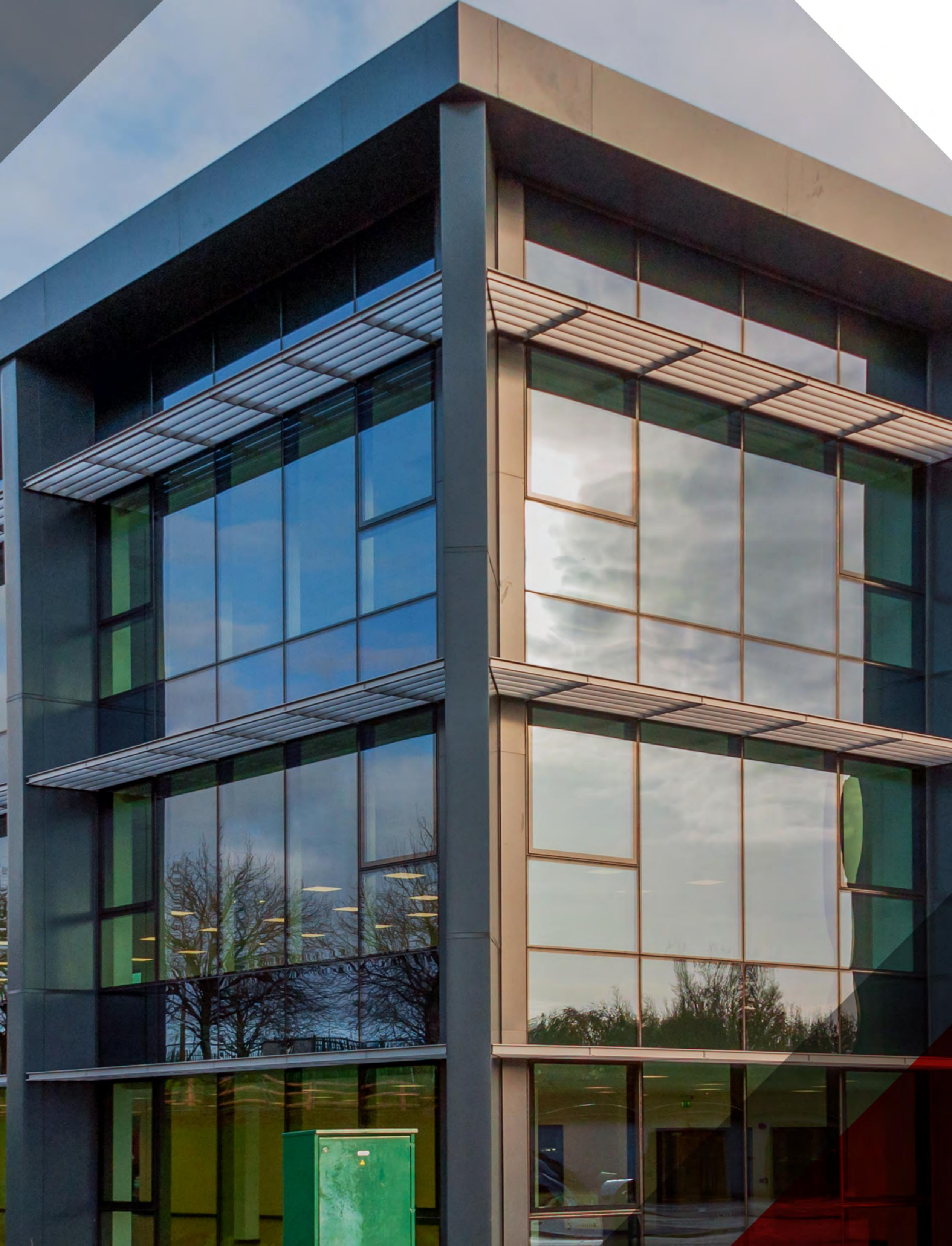
**ALUMINIUM SOLAR SHADING SYSTEM WITH VERTICAL & HORIZONTAL BLADES**
